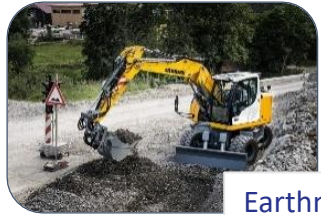
Earthmoving Source: Liebherr
